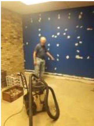
Sept 21 - Ernie repairing walls
